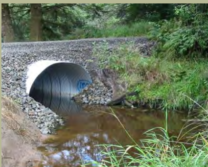
Restoration work replaces old culverts with ones that allow juvenile and adult salmon to migrate both upstream and down.
