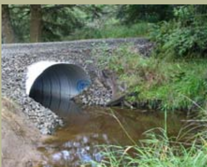
Restoration work replaces old culverts with ones that allow juvenile and adult salmon to migrate both upstream and down.
